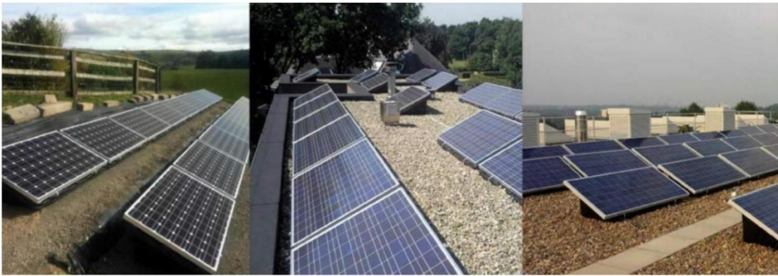
Figure4(c). Finished installation
